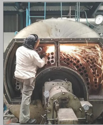
BOILERS REFURBISHMENT & OVERHAUL
