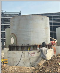
STORAGE TANKS REPAIRS & MAINTENANCE
