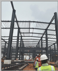
STRUCTURAL STEEL FABRICATION & ERECTION
